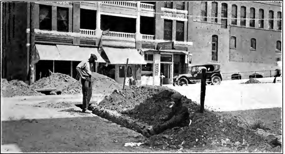
A TYPICAL SCENE IN PRESCOTT WHEN GAS AND WATER MAINS WERE BEING LAID OR RENEWED PRIOR TO PAVING BUSINESS STREETS
